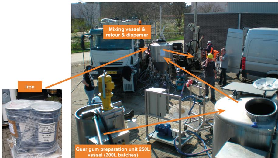
Figure 4. Injection of guar gum stabilised microscale ZVI via direct push
